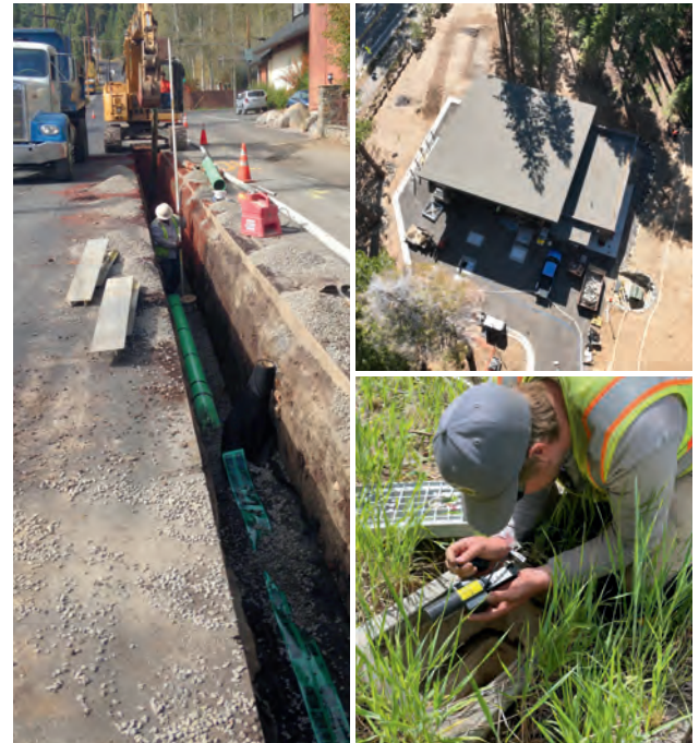
Left: Crews install new sewer main. Top right: An aerial view of the new West Lake Tahoe Water Treatment Plant. Bottom Right: TCPUD staff install a new SMART water meter.
